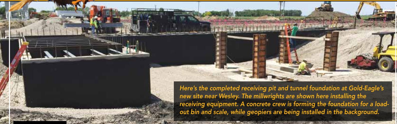
Here's the completed receiving pit and tunnel foundation at Gold-Eagle's new site near Wesley. The millwrights are shown here installing the receiving equipment. A concrete crew is forming the foundation for a load-out bin and scale, while geopiers are being installed in the background.
