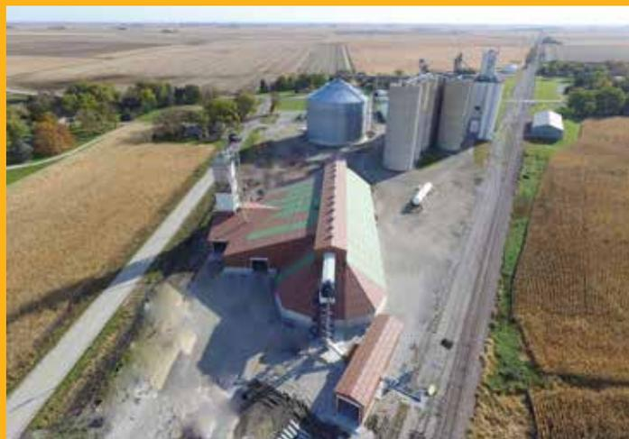
Gold-Eagle's Hardy fertilizer plant is close to completion and will be ready for the 2020 spring agronomy season. This plant has a capacity of approximately 24,000 tons, depending on the densities of products used.
